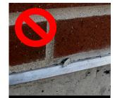
The flashing will pop the mortar out and ooze if the flashing is <u>NOT</u> cut back 1/2" to 1".
