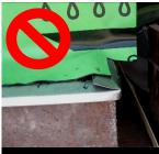
S.S. drips must be prepared such that any over laps are flat. This edge will never seal and water will get under flashing.
